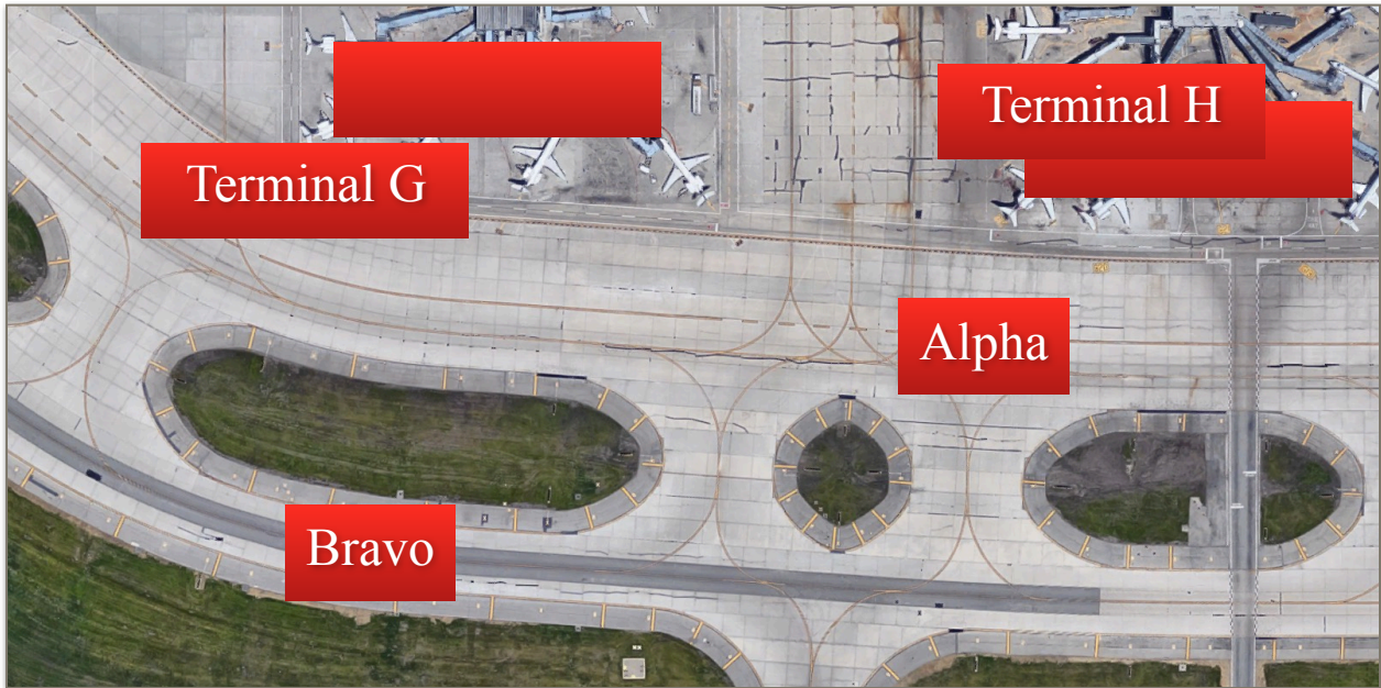
Figure 6. Perimeter Taxiways at ORD Airport. These taxiways are Designated “Alpha” (inner taxiway) and “Bravo” (outer).
