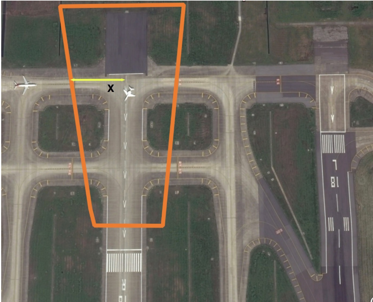
Figure 2. SHA International Airport: North Side.
