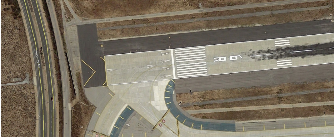
Detail of Departure End of Runway 24L at LAX Airport. Note the 335 foot Displaced Threshold.
